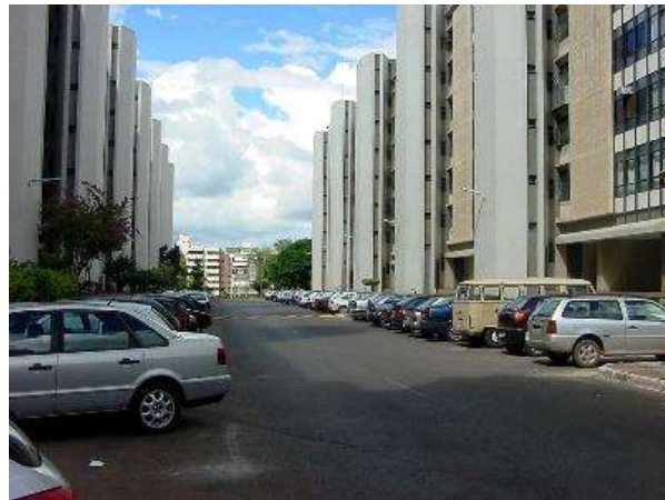
Figure 11 The arid space for vehicles circulation and parking. (Source: the Author.)
